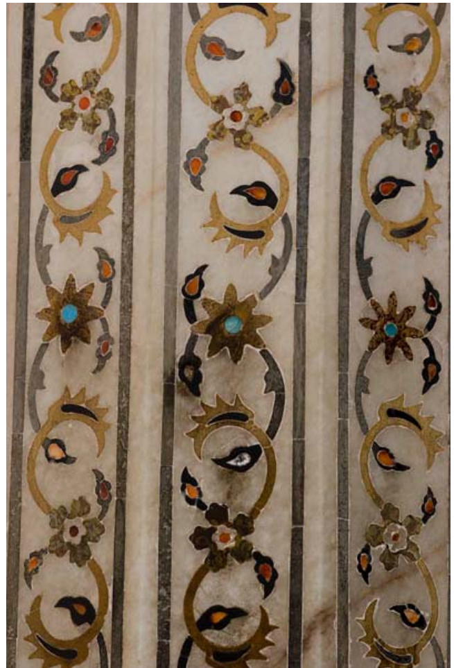
Detail of marble inlaid with semiprecious stones in the Red Fort, Agra.
