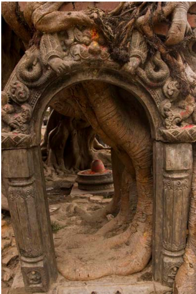
Siva temple overgrown by a tree, Gokana Mathadev Temple, Kathmandu Valley.
