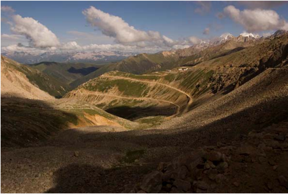
Switchbacks descending from the 5050 m pass on the road to Dege.
